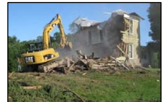
Kenwood Parcel farm house being torn down (J. Parker).
