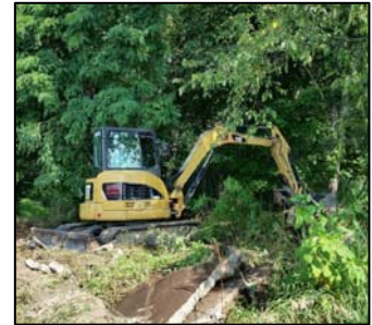
Clean up in process (John Parker).
